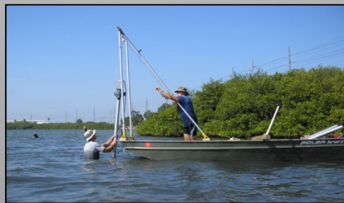
A Vibecore-D coring rig was used to collect eleven 6-foot sediment cores within the project site.
